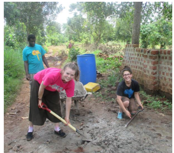
Godfrey, Corrine, and Niomi Mixing Concrete ▶
