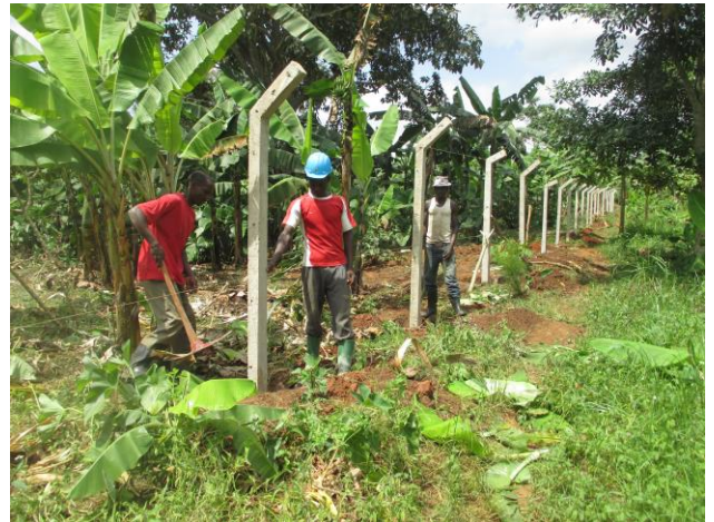
▲ Men working on the fence.
